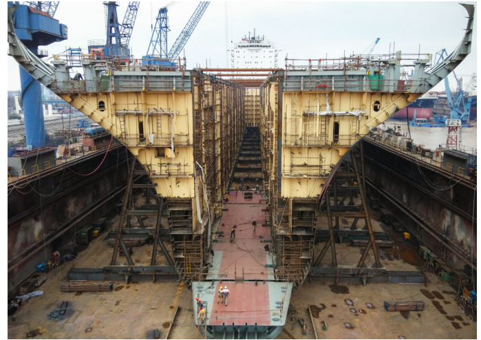
The widening work underway on MSC Geneva .
