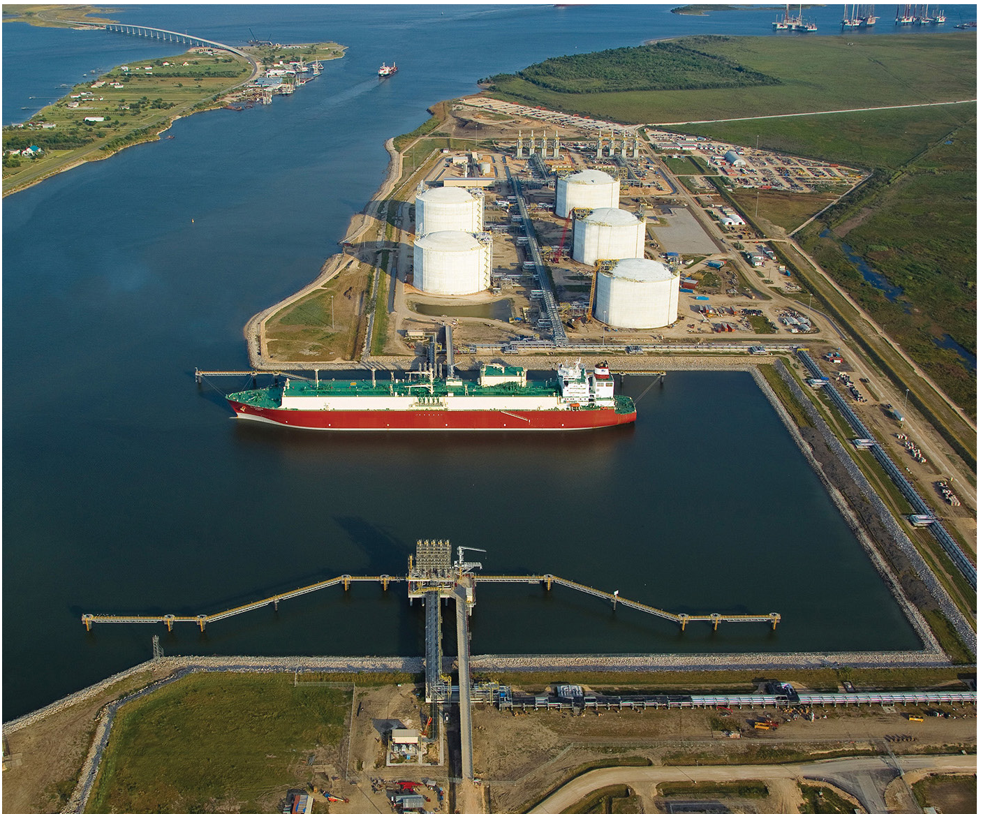
ExxonMobil is working on a $1bn project to convert the LNG regasification terminal at Golden Pass, Texas, into an LNG export terminal.
